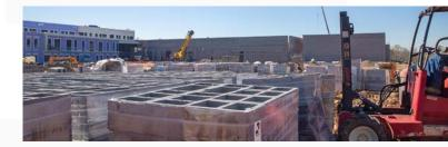
thermal mass, or its ability to absorb and hold heat. This trait allows CMUs to hold in cool air in the summer months and radiate warm air in the winter month, helping to keep the inside temperature steady while the outside temperature rises and falls.
